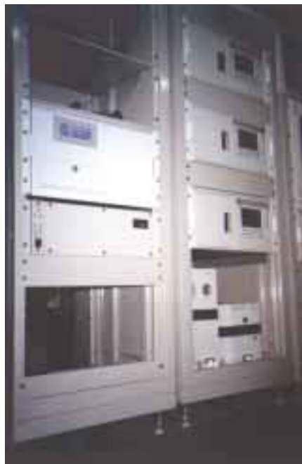
Full-automatic Ambient Air Monitoring System (NO x , SO 2 , SPM, CO and meteorological data are gathered and processed.)
