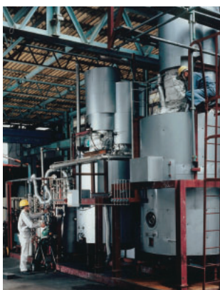
The CO 2 fixation technology demonstration plant that produces reusable carbon nanofibers.
